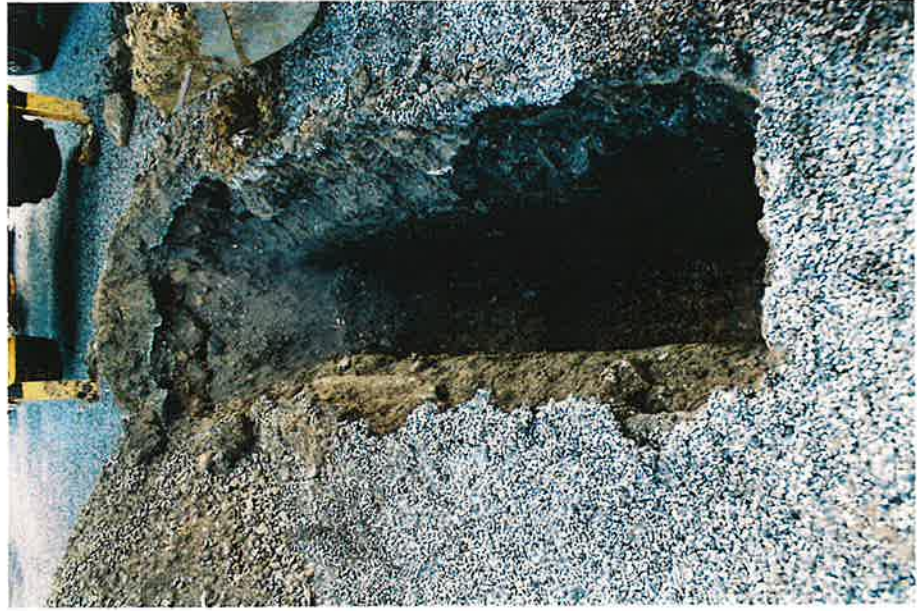
Plate 2: Trial pit 5 from west (05_06_CPI_21)
